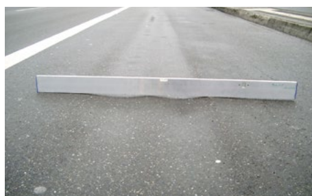
At high temperatures and under high loads resulting from e.g. heavy goods vehicle traffic, asphalt is deformed and ruts develop. (Photo: KIT/ISE)
