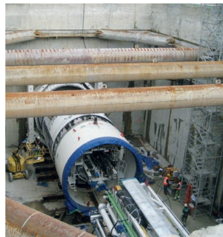
Assembly of the tunnel boring machine in the DESY starting shaft in Hamburg, 2010. (Photo: P. Kudella, KIT)
