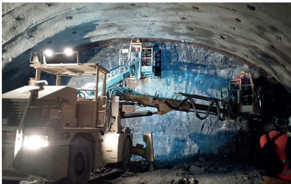
Drilling blast holes to advance the roof section of the Brenner Base Tunnel in 2015. (Photo: P. Kudella, KIT)
