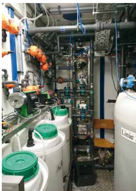
Ultrafiltration pilot plant at the Steinhäule sewage treatment plant in Neu-Ulm. (Photo: Dr.-Ing. Johannes Alexander, IFG)
